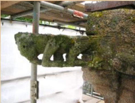
Fig.: 16-17.: Gargoyle before and after cleaning and conservation. Phosphor bronze armatures were applied to support the fragile stone.
