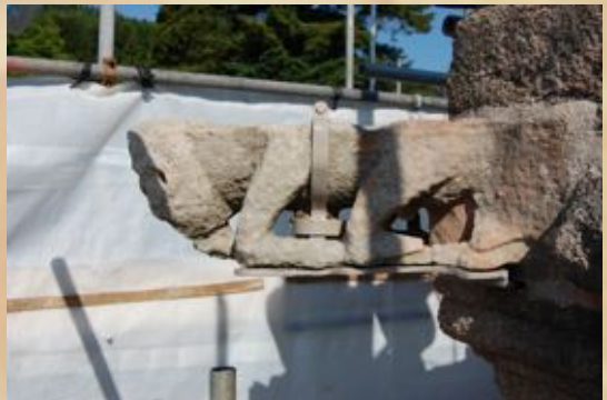
Fig.: 16-17.: Gargoyle before and after cleaning and conservation. Phosphor bronze armatures were applied to support the fragile stone.
