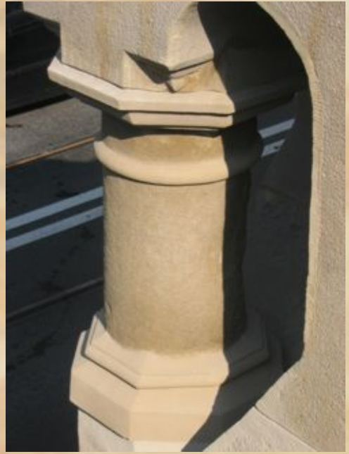
Fig.: 26, 27.: Cracow; Reconstructions made using stainless steel armatures and two ready made mixes by Baunit and Remmers, upper part mixed with Remmers Haftfest for better adhesion.
