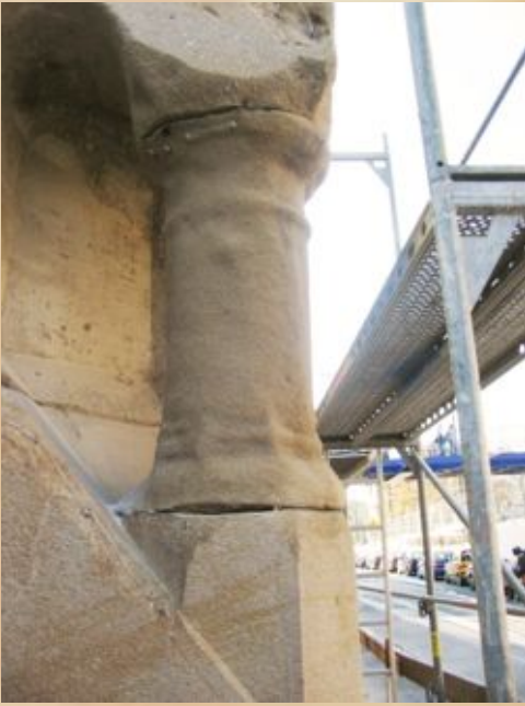
Fig.: 26, 27.: Cracow; Reconstructions made using stainless steel armatures and two ready made mixes by Baunit and Remmers, upper part mixed with Remmers Haftfest for better adhesion.
