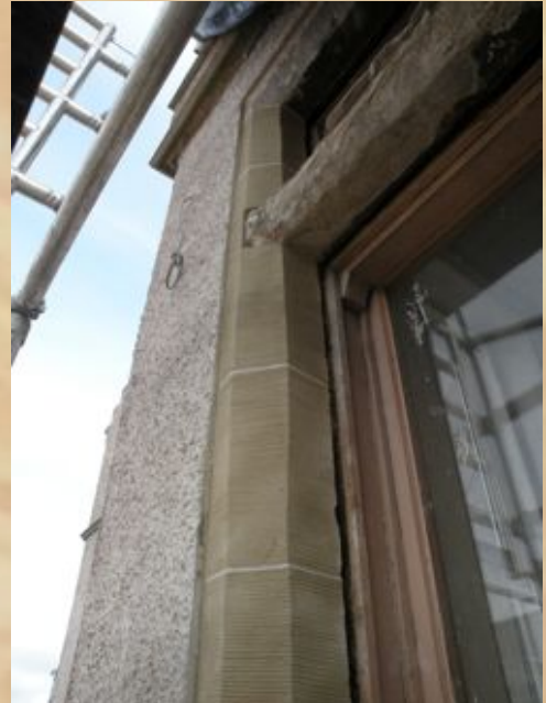
Fig.: 28, 29.: Nairn; Reconstruction based on Lithomix. Repair was matched to the new stones replacing the transoms and mullions.
