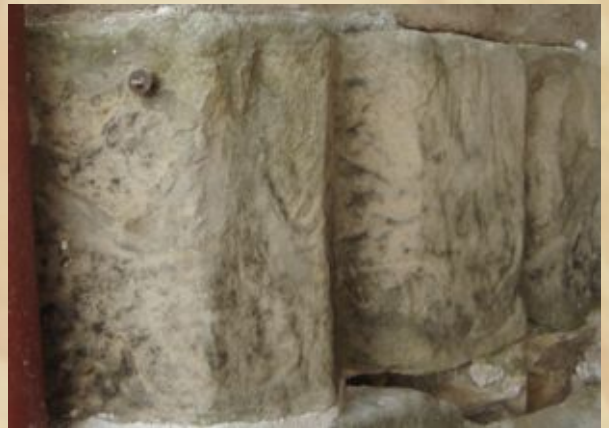
Fig. 68-72.: Responsible for lime mortar repairs on the Crown Tower of King's College . Leading a small group of conservators.
