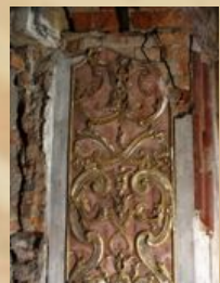
Fig. 55- 59.: The chapel was seriously damaged during second World War and also because of the fire in XIX century. Most of the stuccos appeared to be hollow and de-attached from the disintegrated plaster and brick wall. Stucco preservation including injections of silanes and grouting. Photographic documentation of the entire chapel form the inside.
