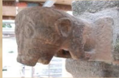
Fig.: 14-15.: Gargoyle before and after cleaning and conservation. Chin of the gargoyle was re-attached.
