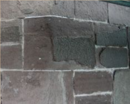
Fig. 76-77.: Dingwall Town Hall Balcony. Conservation of the main part. Report with recommendations how to proceed with each stone, Steam cleaning, removal of old resin repairs, consolidation of delaminations, acrylic mortar and lithomix repairs, inserting stainless steel armatures into delaminating stones.
