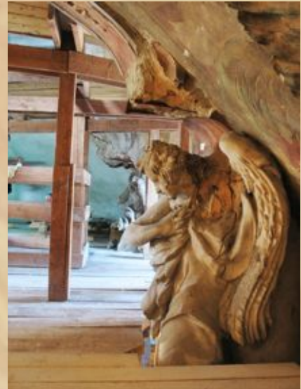
Fig. 55- 59.: The chapel was seriously damaged during second World War and also because of the fire in XIX century. Most of the stuccos appeared to be hollow and de-attached from the disintegrated plaster and brick wall. Stucco preservation including injections of silanes and grouting. Photographic documentation of the entire chapel form the inside.
