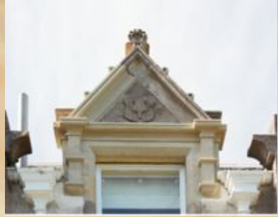
Fig. 1-2.: One of the pediments: pediment with shield and stags head. Before and after conservation. (Stones cut by the stone mason)
