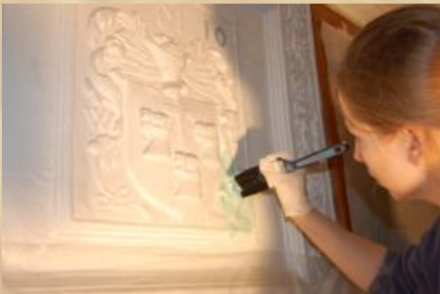
Fig. 38-39.: Making the mould and casting the copy of one of the plaster decorations.
