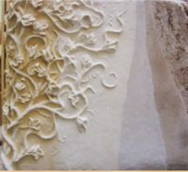
Fig. 86.: Example of pargeting. Made using lime mortar and then limewashed.
