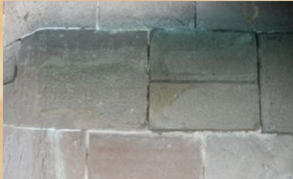
Fig. 76-77.: Dingwall Town Hall Balcony. Conservation of the main part. Report with recommendations how to proceed with each stone, Steam cleaning, removal of old resin repairs, consolidation of delaminations, acrylic mortar and lithomix repairs, inserting stainless steel armatures into delaminating stones.
