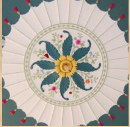
Fig.: 78,79.: Crack consolidation and re-painting of the damaged ceiling rosetta.
