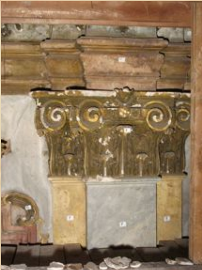
Fig. 55- 59.: The chapel was seriously damaged during second World War and also because of the fire in XIX century. Most of the stuccos appeared to be hollow and de-attached from the disintegrated plaster and brick wall. Stucco preservation including injections of silanes and grouting. Photographic documentation of the entire chapel form the inside.
