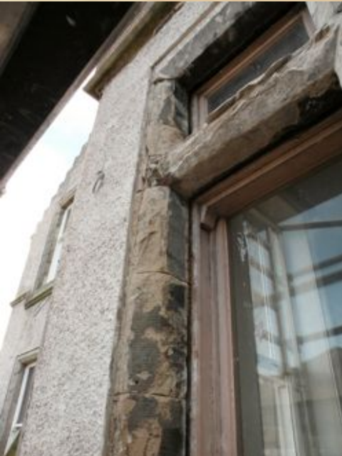
Fig.: 28, 29.: Nairn; Reconstruction based on Lithomix. Repair was matched to the new stones replacing the transoms and mullions.
