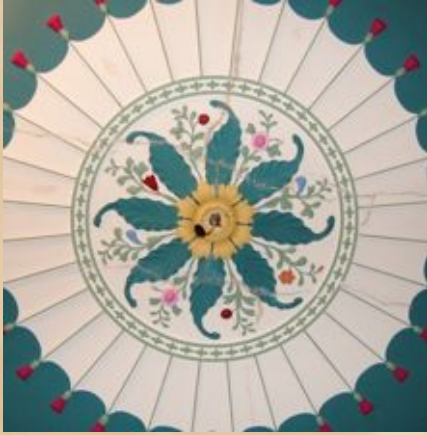
Fig.: 78,79.: Crack consolidation and re-painting of the damaged ceiling rosetta.
