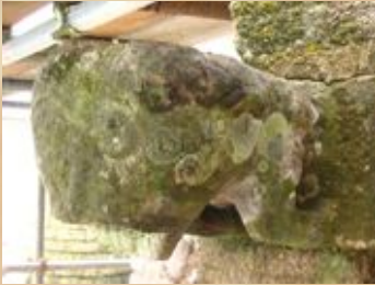
Fig.: 14-15.: Gargoyle before and after cleaning and conservation. Chin of the gargoyle was re-attached.
