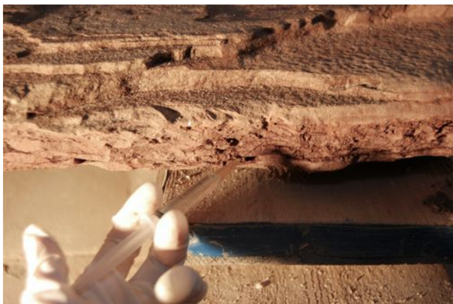
Fig.: 8. Consolidation with solutions of Paraloid B72.
