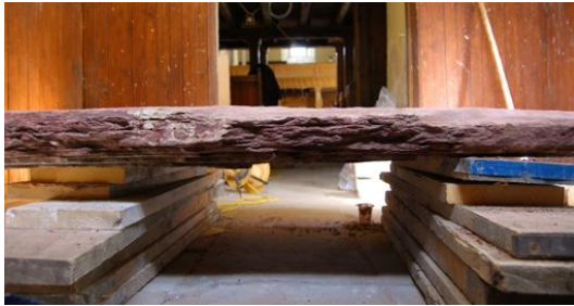
Fig.: 10. In the middle of acrylic mortar repairs. Left hand side- after mortar repairs. Right hand side – before repairs.
