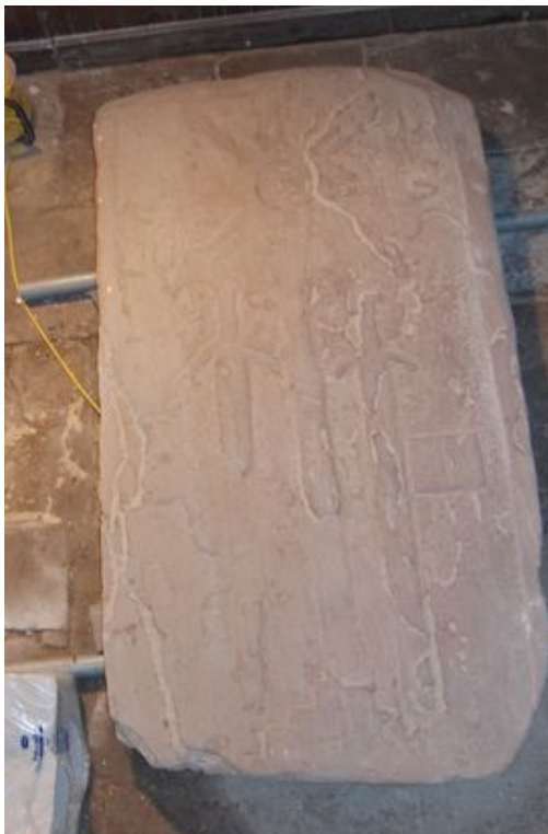
Fig.: 1-2. Tombgrave before conservation. Efflorescence (crystalised salts) is visible on the left hand side of the stone.
