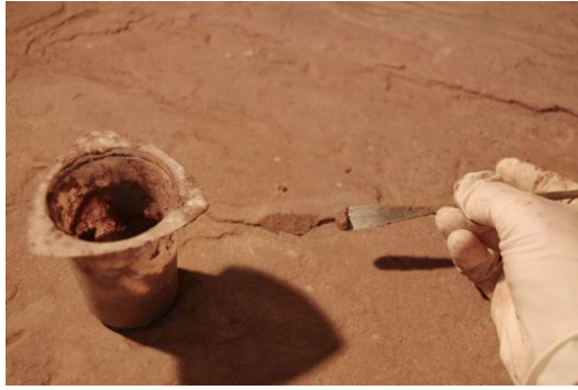
Fig.: 9. Acrylic mortar repairs.
