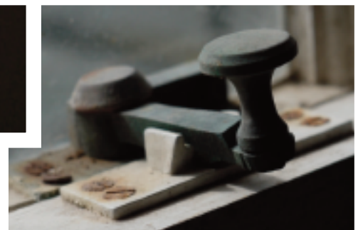
joining new wood with the old
