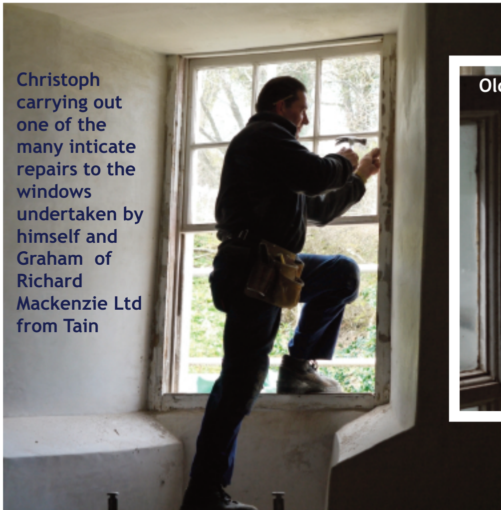
joining new wood with the old
