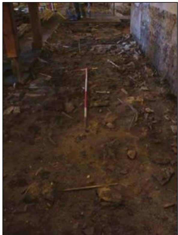
Plate 16 East aisle, after removal of wooden floor, before excavation
