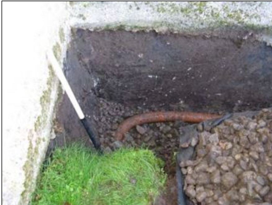
Plate 1 Corner of E wall and E porch, by door, showing bitumen, cement harl and perforated pipe drainage as found
