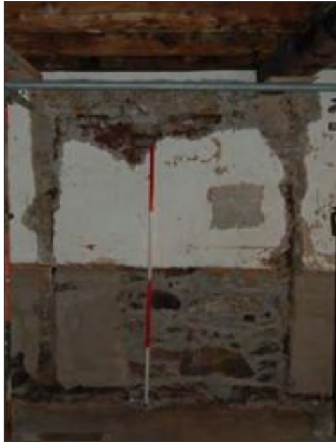
Plate 7 Blocked doorway (interior view)
