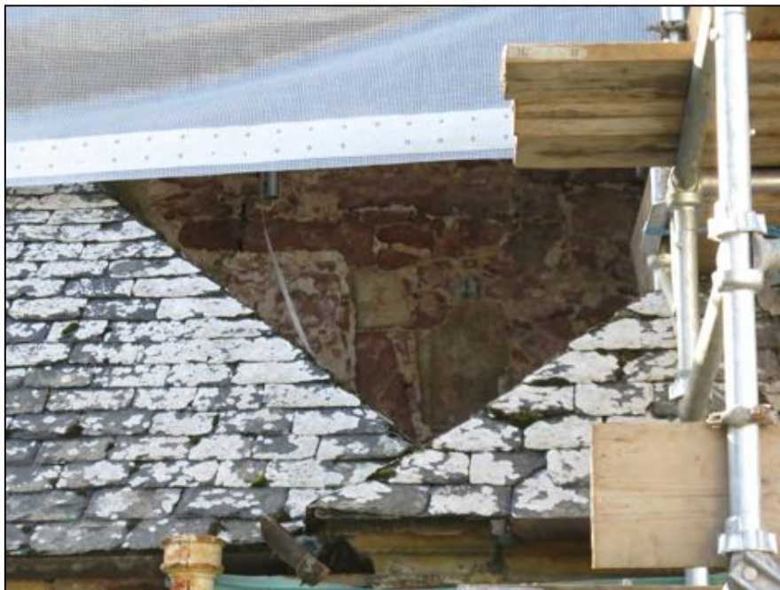
Plate 10 Evidence of blocked 16 th c. window in E gable, largely hidden by E porch and vestry
