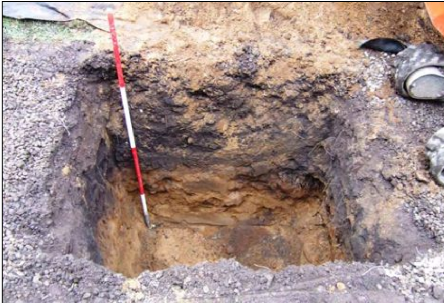
Plate 3 Soakaway in churchyard
